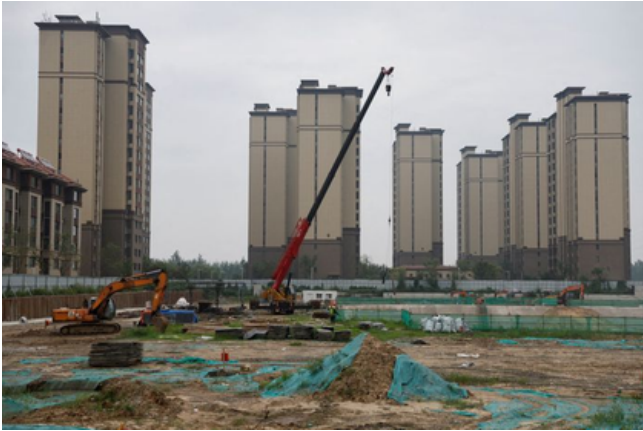
A Country Garden development under construction. Source: Reuters
